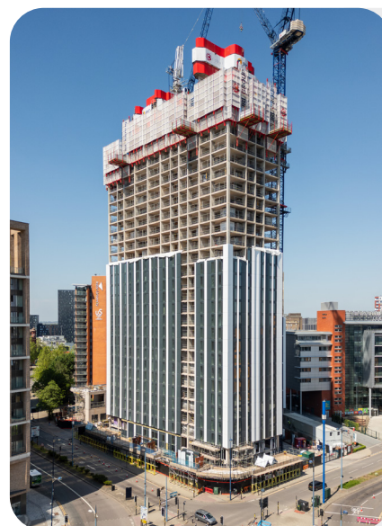
One Eastside in Birmingham is providing around 300 jobs during construction.
